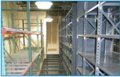
Rack & Shelf-Supported Catwalk Mezzanine (Single-Level)
