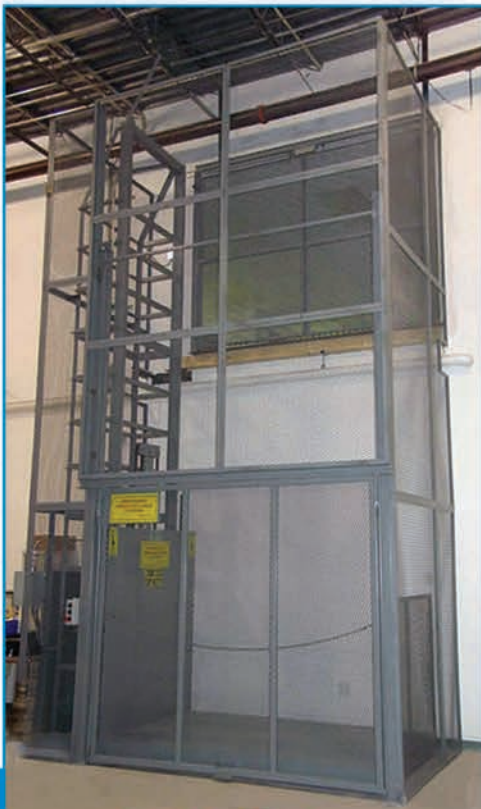
Wire Mesh Shaftway (Not Fire Rated)
