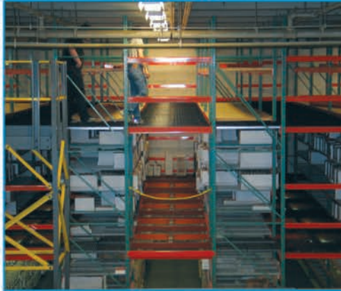
Rack-Supported Catwalk Mezzanine (Two-Level)
