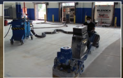
Surface Preparation and Concrete Repair
